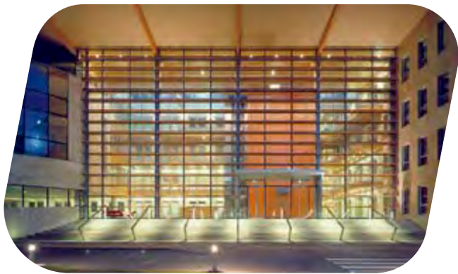
Pilkington Optilam ™ Therm 8,8 – Tulipan House office center, Warsaw, Poland
