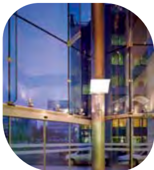
Pilkington Planar ™ – Crown Tower office centre, Warsaw, Poland
