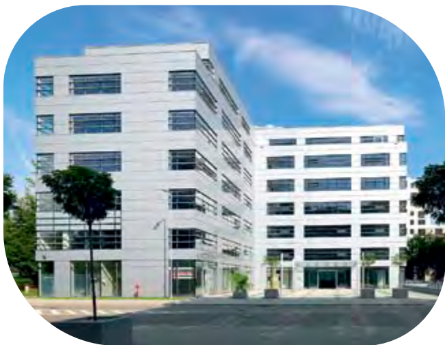
Pilkington Optifloat™ Clear – Luminar, Warsaw, Poland
