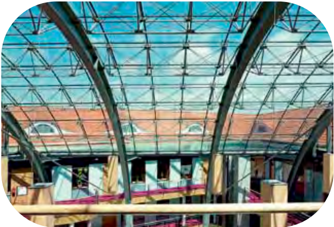
Planar ™ | SentryGlas ® System – Times office centre, Wrocław, Poland
