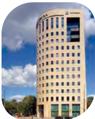
Pilkington Insulight™ Sun – Królewska office center, Warsaw, Poland
